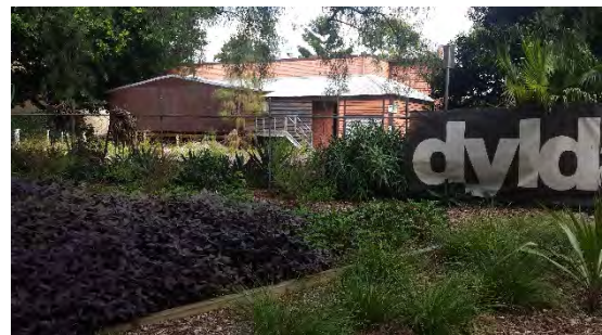
Photo 26 – The eastern site of the building facing west
