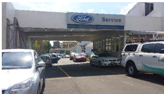
Photo 6 – The Ford service workshop fronting Dixon Street facing north with potential UST and bowser to the north of canopy area
