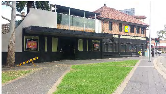
Photo 20 – PJ's Irish Pub facing south west from Parkes Street
