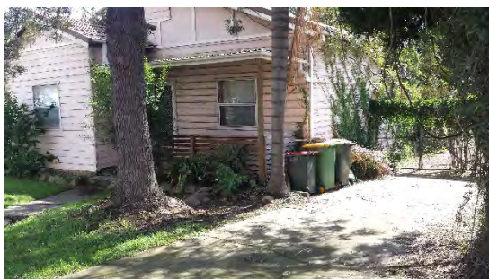
Photo 5 – Residence fronting Dixon Street facing north
