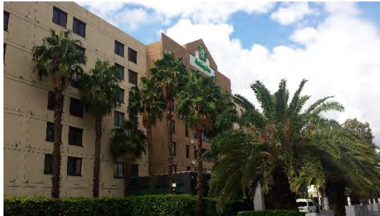
Photo 27 – The Holiday Inn Hotel facing south east from Anderson Street
