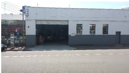
Photo 32 – The southern portion of the warehouse building fronting Marion Street facing north
