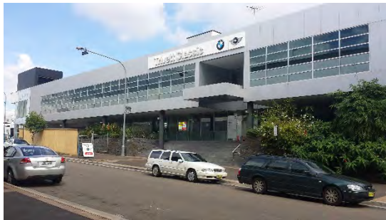
Photo 23 – Trivett Classic BMW and Mini show room building
