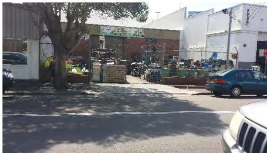
Photo 31 – Street view of the warehouse building fronting Marion Street
