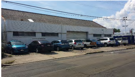
Photo 16 – Warehouse building with Super Six roofing fronting Boundary Street
