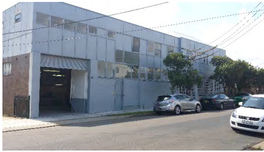
Photo 10 – Warehouse style building fronting Rosehill Street facing north
