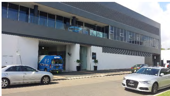
Photo 29 – The Trivett automotive service centre building facing east from Anderson Street
